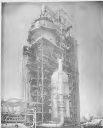
Nearly Completed, New Reactor Glimpses In the Sun.
